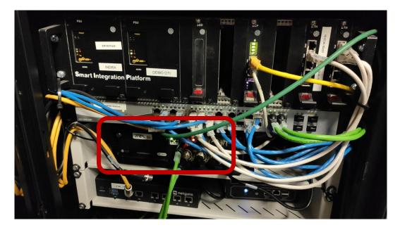
Figure 82 ACS integrated into INDRA's rack
